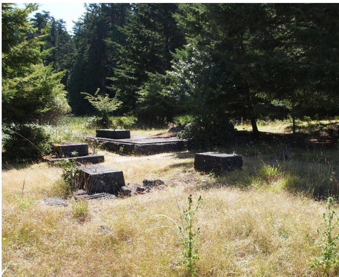
FIGURE 1. Boatyard machinery foundations.
