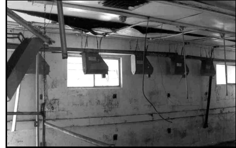
Figure 7-5 – Remnants of the milking apparatus in 1998
